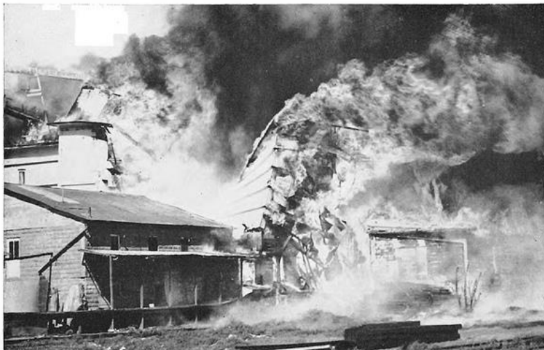
Flour dust explosion, Hutchinson, Kan., May 1, 1947. — Improper training of employees for fire emergencies was responsible for the disastrous explosion. Instead of calling the fire department on discovering a belt fire, employees attacked the blaze with solid stream extinguishers and pails of water, thereby stirring up dust that exploded.
